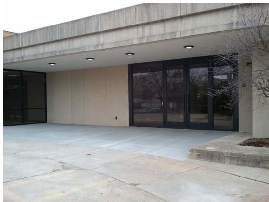
The Synagogue's new front entrance; to the left is one of the new floor-to-ceiling windows installed in our new library.
